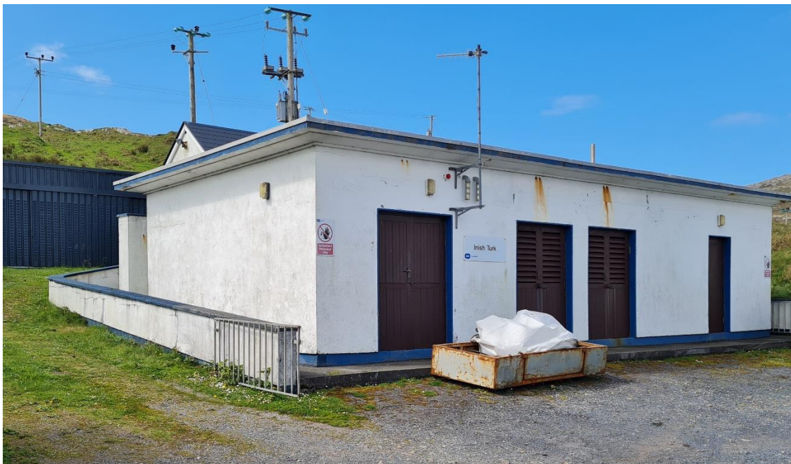
Figure 3: Generating Station Inishturk (housed generators in grey building in background)
